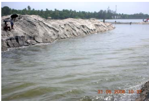
Thottappally Pozhi cut open D/S of Spillway
